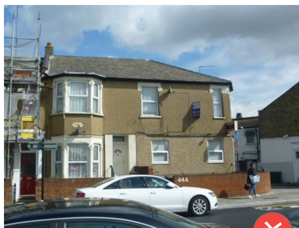
Brickwork should not be painted or covered with render, pebble-dash or cladding.
